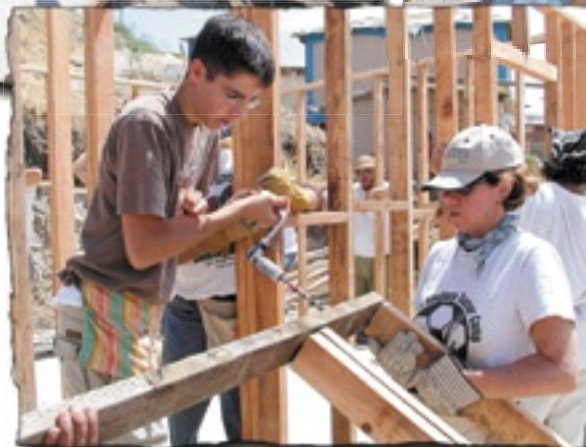
Day 2 (right): Wood is measured, cut and assembled to create the walls. All the tools (except for the cement mixer) and hand tools, and even team members with no prior experience in construction quickly catch on!
