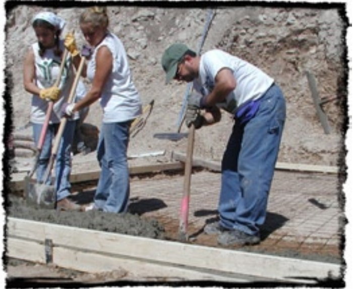
Day 2: George Dickos pulls support wires up into the thickening cement.
