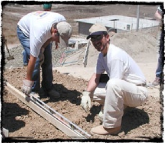
Day 2: Father John helps measure boards for the concrete form.
