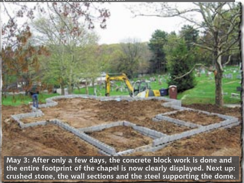
April 29: As the concrete blocks are laid, the shape of the building begins to quickly appear. The view here is looking over the altar (the curved section) into the church.
