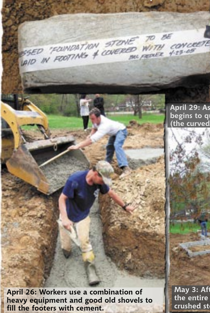
April 25: The stone laid at the "Laying of the Foundation" service was placed in the center of the excavation before the cement foundation was poured.
