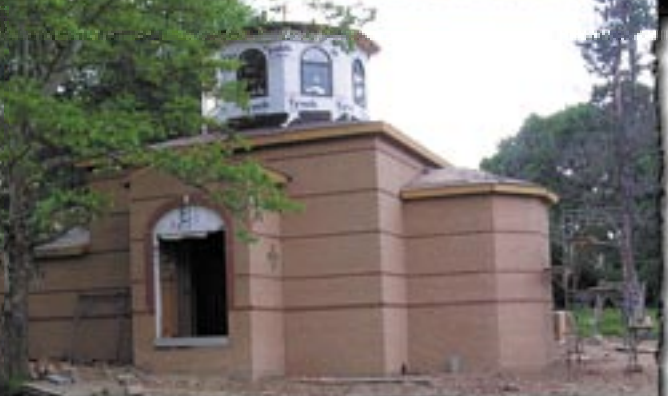
June 2 (left): The bricklayers begin at the front right corner. June 20 (above): The southeast walls are the first to be completed. The curved section to the right is where the altar will be located, facing east according to tradition.
