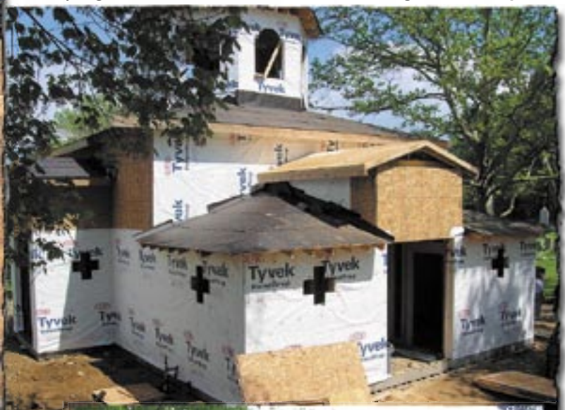
May 17 (left): Looking in what will become the front door, with the dome starting to take shape on top. May 21 (below): The exterior skin is nearly complete and ready for the bricklayers to begin. The Cross-shaped holes are for glass-block windows, which will add security, light and even a small touch of Pittsburgh to the chapel!
