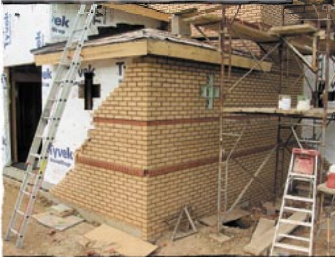
June 2 (left): The bricklayers begin at the front right corner. June 20 (above): The southeast walls are the first to be completed. The curved section to the right is where the altar will be located, facing east according to tradition.
