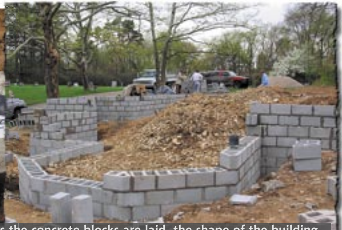
April 29: As the concrete blocks are laid, the shape of the building begins to quickly appear. The view here is looking over the altar (the curved section) into the church.
